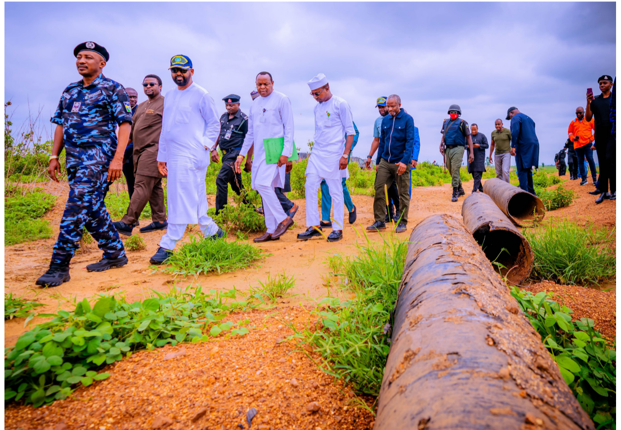
NNPC Ltd with other stakeholders during the inspection of the vandalised crude oil pipeline.
